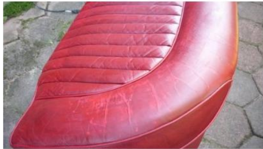
1 st coat of dye added
