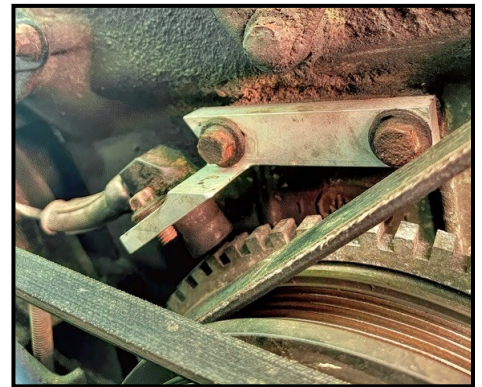
The Andy Bracket Installed
