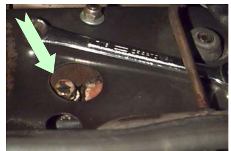
Fig.2—Close-up of vent
