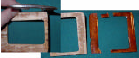
Vent panels after removal
