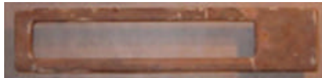
Center vent after repairing with plastic wood; an example of the first stages of restoration.
